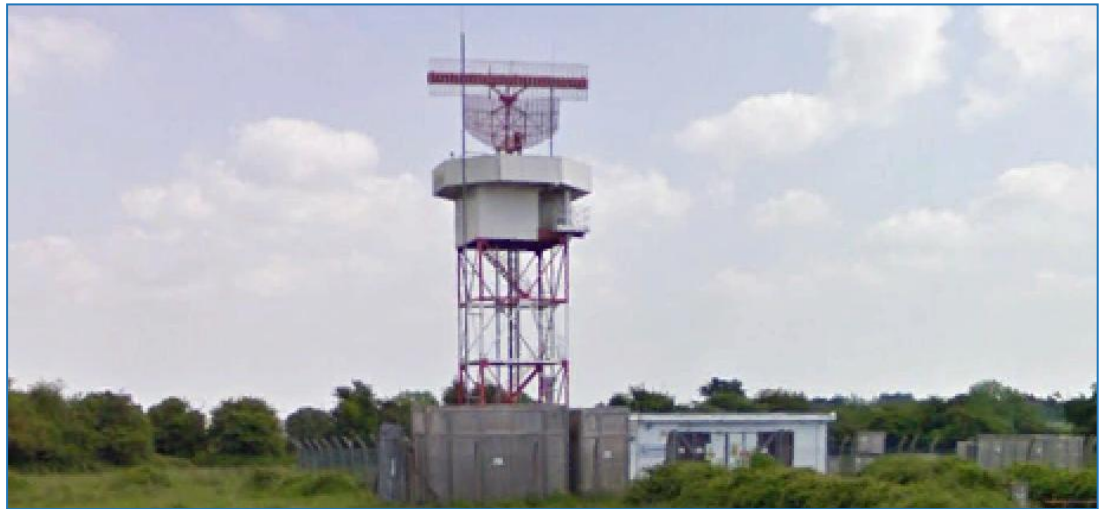
Figure 2: Shannon Airport PSR with co-mounted MSSR
