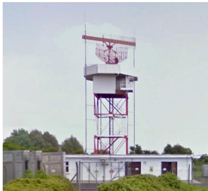
Figure 3.3 The combined PSR and Mode-A/C MSSR at Shannon International Airport (Image source: Street View).
