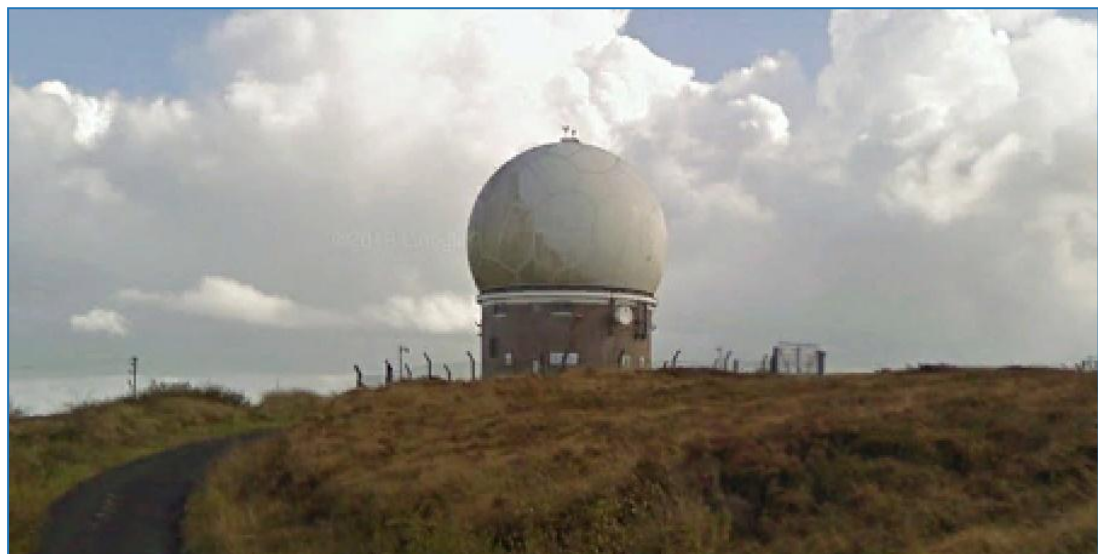
Figure 6: Woodcock Hill MSSR system
