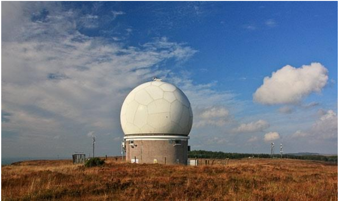
Figure 3.3 The stand-alone en-route Mode-S MSSR at Woodcock Hill housed in a radome (Image source: IAA).
