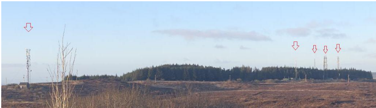
Figure 25 The telecoms masts at Woodcock Hill one of which was identified by AirNav causing deflections of the radar beams from the Woodcock Hill MSSR ( photo taken with back to the MSSR )
