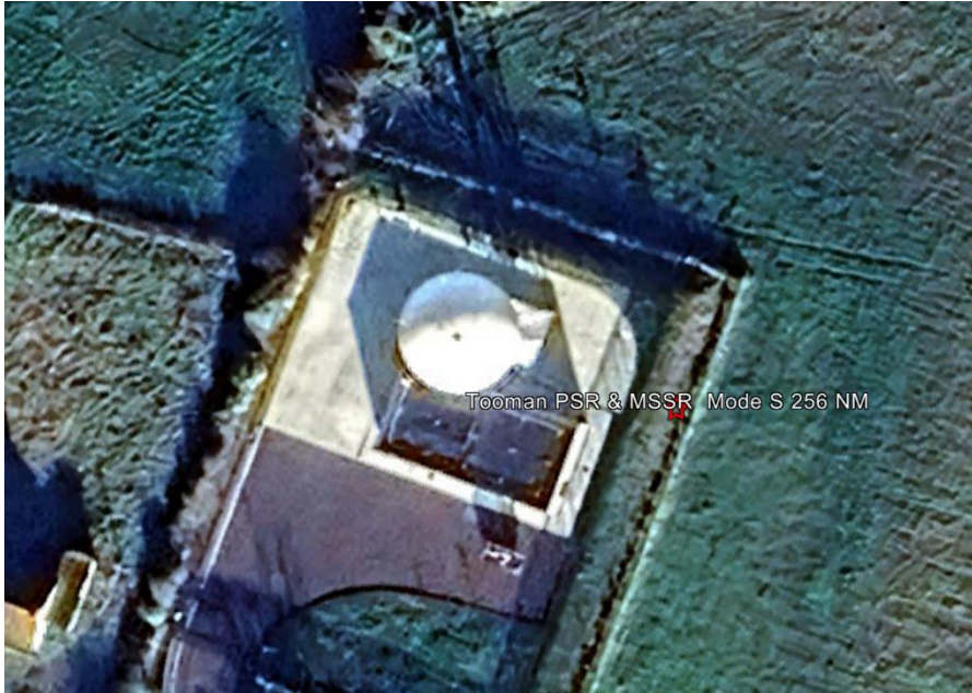
Figure 4.37 The combined PSR and en-route MSSR at Tooman Hill housed in a radome. Note that the provided coordinates are slightly off (Image from Google Earth).
